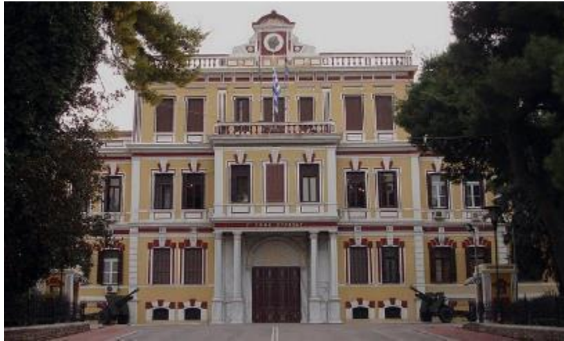
Fig. C.6 3rd Army Corps building
