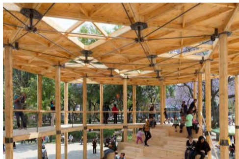
Internal CLT Timber Structure for Exhibition Halls
