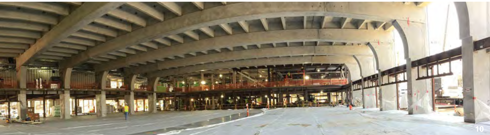
Picture 10: Long span modular concrete floor plate system
