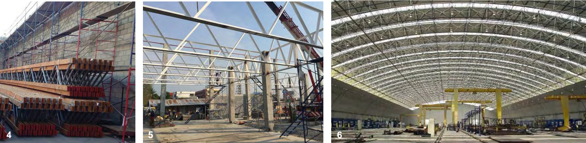
Picture 7-9: Modular glue lam timber systems
